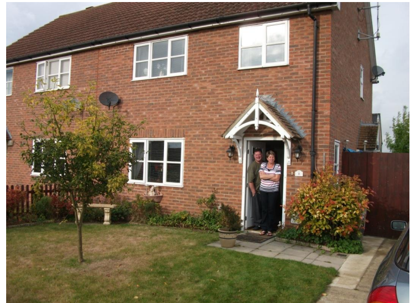
Right: GSHP installed in 2012 Coil buried in front garden
