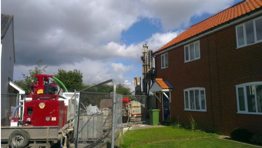
Above: Drilling rig
